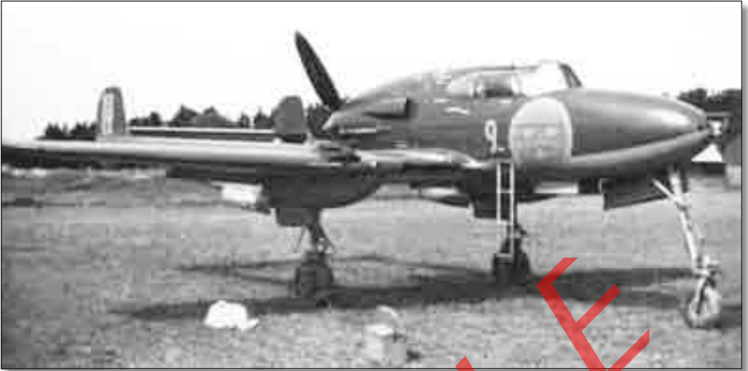
Another F9 Wing J 21A, this machine nicely demonstrates the truncated '9', as well as the retractable, telescopic boarding ladder. The muzzle of the starboard boom-mounted 13.2-mm machine-gun is also prominent. (Via the Hallind-Group)
