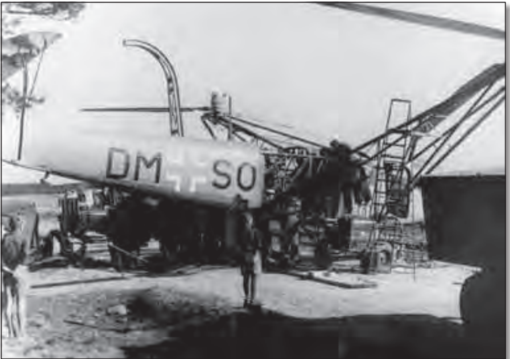
Fa 223 Drache V11 DM+SO during an engine exchange in the field.
