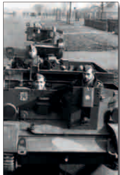
so are often difficult to spot in photographs. This Universal Carriers of this Czech unit in UK around 1942 have the SLING HERE (or possibly LIFT HERE) instructions stencilled next to the front lifting eyes - the same is almost certainly the case at the rear. Note the gas detector paint on the front. (B. Kudlička coll.)
